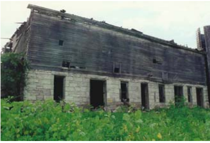
100-year-old barn dismantled for lumber & stone
