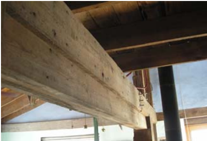
Barn beams provide supporting structure for house
