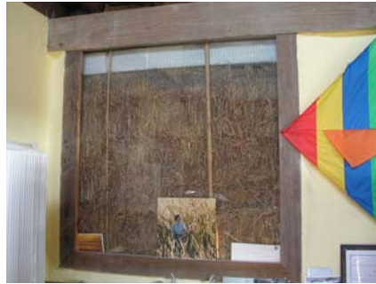
"Truth window" shows Indiagrass bales & construction technique
