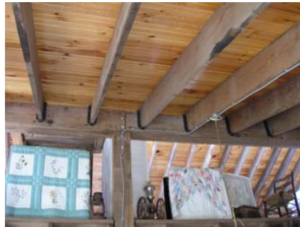
View up into loft from kitchen
