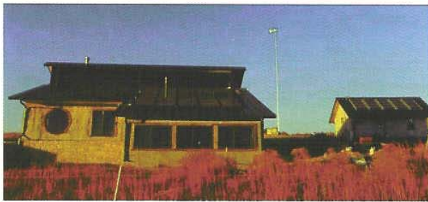
Women's PV Workshop participants used solar power alone to build Jane Koger's straw bale house, located in rural Kansas.
